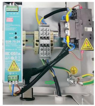
The power cable for the 230 VAC is connected to the terminals inside of the cabinet, as shown in the picture on the left.
